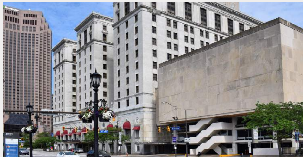
G - W 3rd & Superior facing southeast
